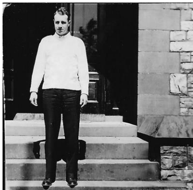
Brad on steps of Conklin Hall, the dormitory at Mont Alto Forest Academy. Mont Alto is in the mountains of south-central Pennsylvania. The Forest Academy was the site of an iron smelter. Water was diverted upstream of campus and channeled into the smelter and then to a series of waterfalls in front of Conklin Hall and into a trout pond. It flowed down a series of manmade falls and into a trout pond. BB By the time Brad attended the Forest Academy it provided only the first year of the forestry program. Students transferred to the main campus to complete their degrees.
